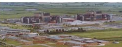
Berkeley Magnox Reactors
